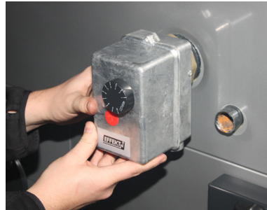
2. Installation of the thermostat
