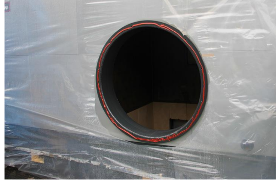
Figure 2 Sealed round shaped burner opening
