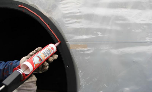
Figure 1 Sealing burner opening with a heat-resistant silicone (also heat-resistant gaskets can be used if available)
