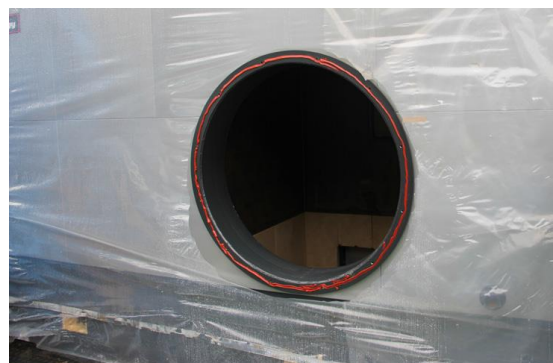
Figure 4. Silicone mass in the burner opening.
