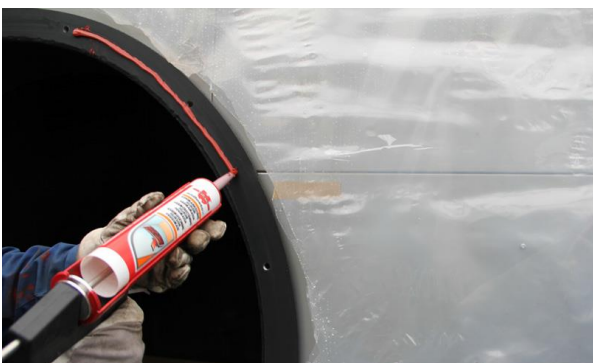
Figure 3. Extrusion of heat-resistant silicone.
